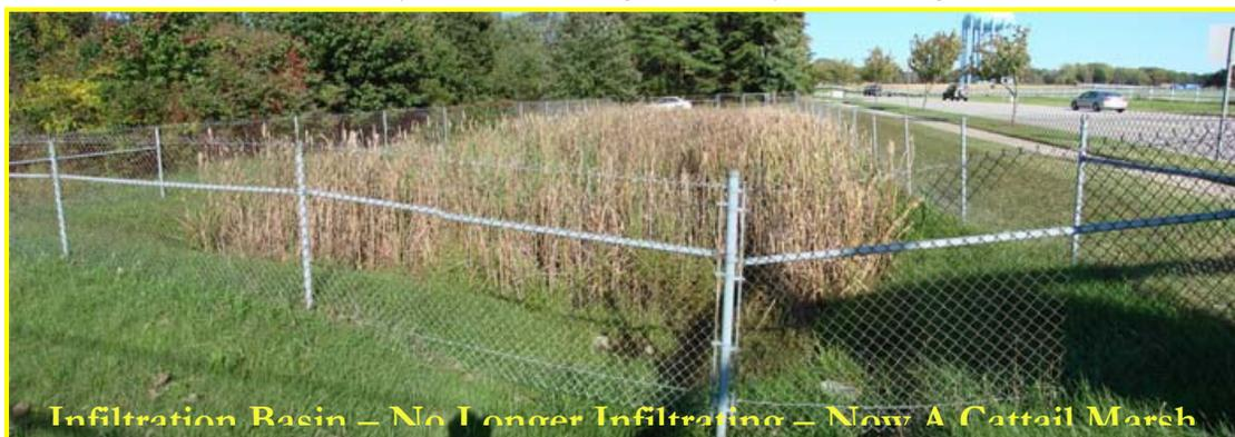
The cattail marsh shown above is an infiltration basin which is no longer functioning. All such facilities sighted had failed. Wet ponds work well, but also need maintenance – if they are partially filled with
