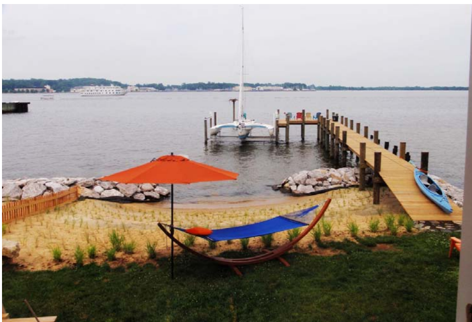
Living Shoreline in place at the conclusion of the Horn Point project.
